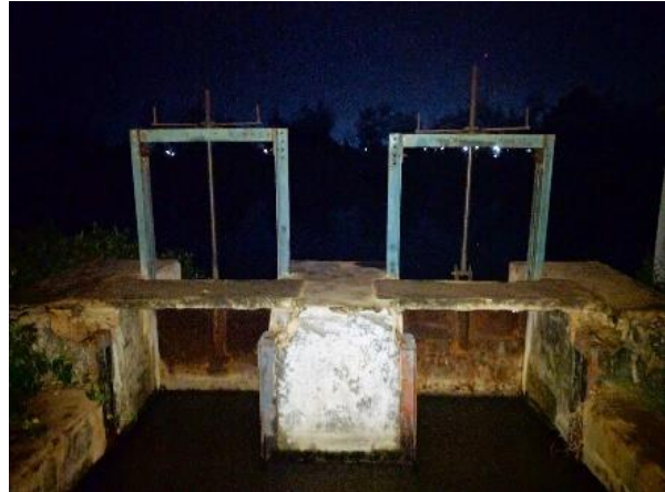
Figure 5, intakes are closed at night when the river Meduri is to high
