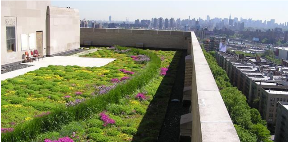
Figure 5 example green roofs
